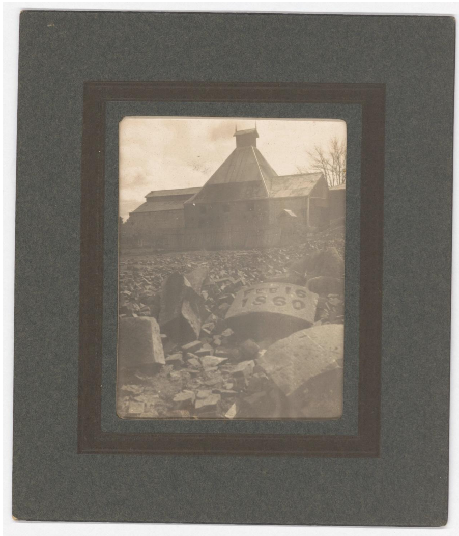
Figure 31: Demolition of the Castlemaine Distillery Co (P662).
